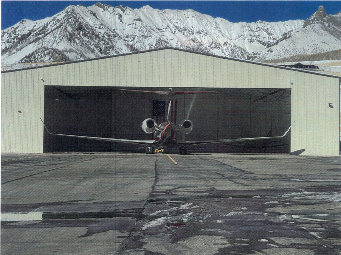
Gulfstream G650 Staged in front of Hangar 29 (3' left/right wingtip clearance) Two wing walkers required for parking in hangar (105' door opening)
